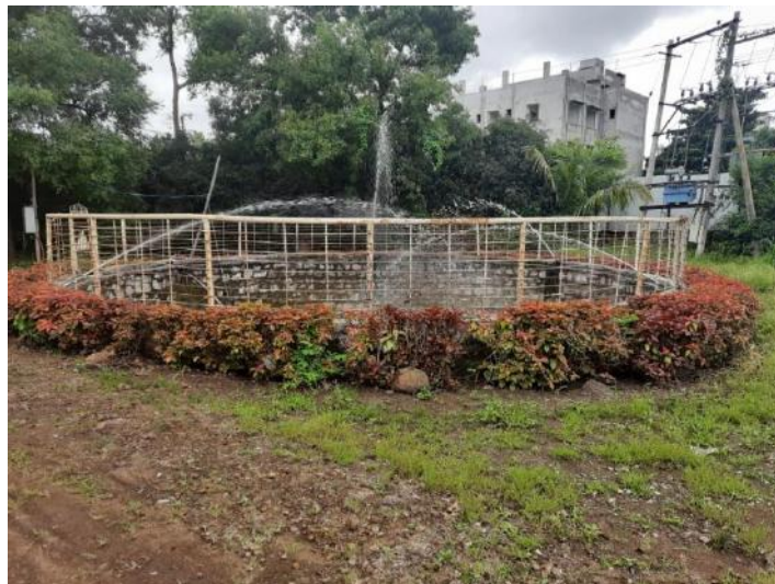
Open well near swimming pool
